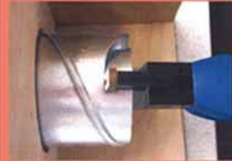
Trimming the duct
