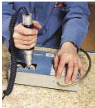
Sampling check of the torque applied in a joint
