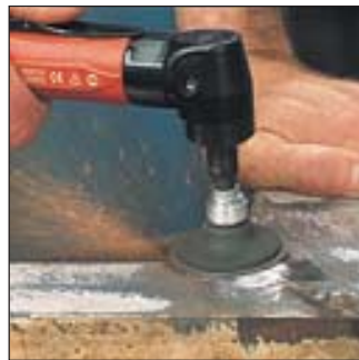
PLANING DOWN WELD
